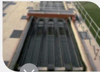
The **MULTIFLO™** process can be used in clarification or water softening applications. It combines the coagulation, flocculation and counter-current lamella settling stages in a single unit.
